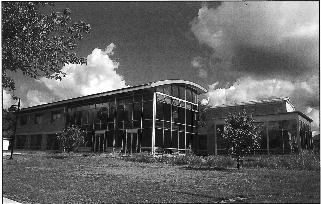
A 60 kW grid-connected photovoltaic array on the roof of Oberlin College's Adam Joseph Lewis Center for Environmental Studies generates a substantial portion of the annual electricity use of the facility.
